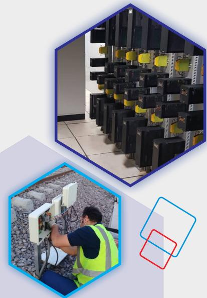
Tuning Unit (TU) consists of lumped passive components, is part of ESJ and connects to the receiver or transmitter by MU. There is a different TU for each frequency, at nominal frequency, TU shows high impedance, passes the signal related to the relevant track, and has a very low impedance at the frequency of the adjacent track.
